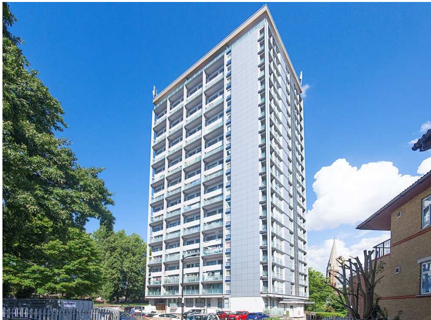
Little Venice tower blocks, Warwick and Brindley estate, 21 storeys
