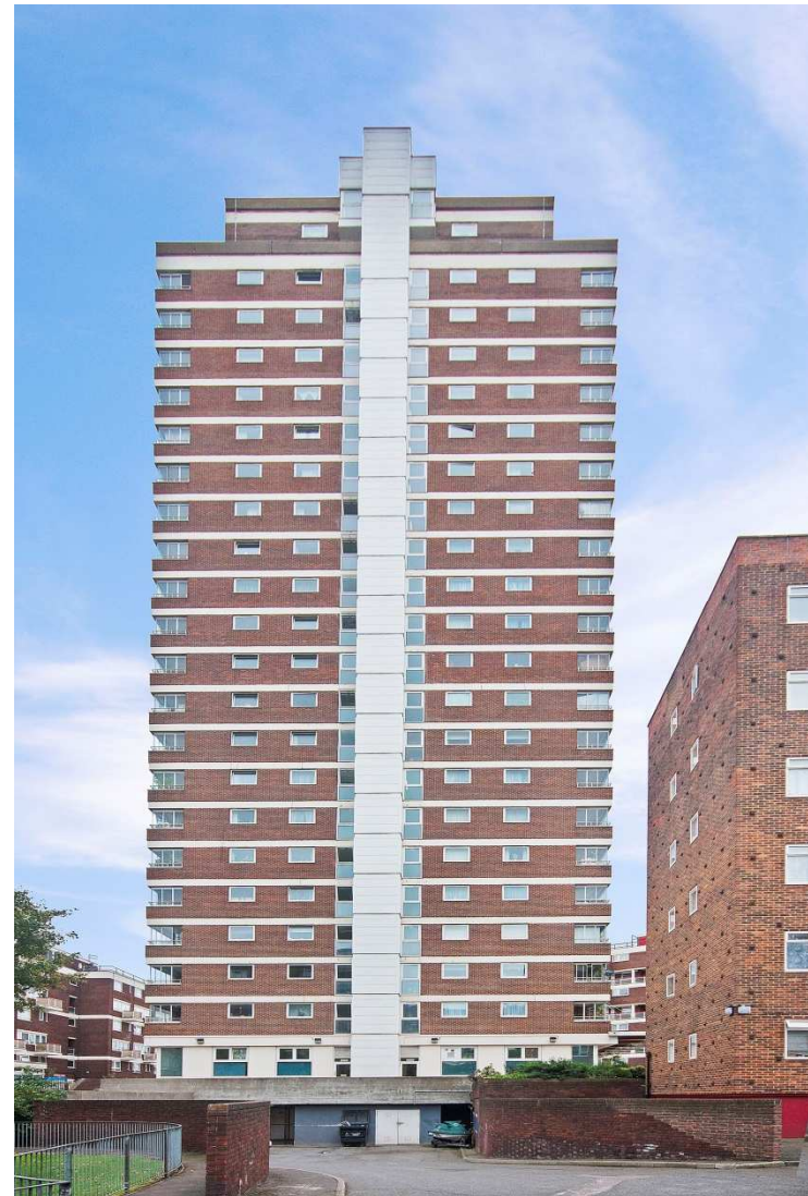
Glastonbury House, supportive housing, Pimlico, 23 storeys
